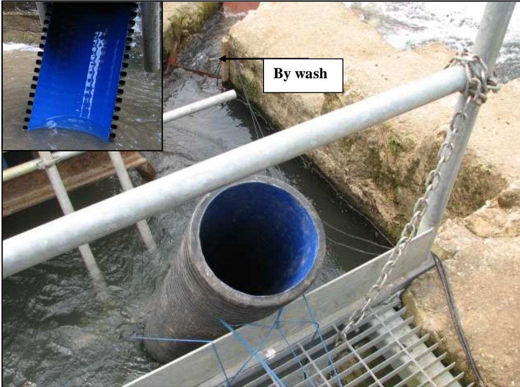
**Figure 2:** photo showing the pipe used to introduce fish to the intake area above the turbine and by-wash, and the escape window at the end of the pipe (inset).
